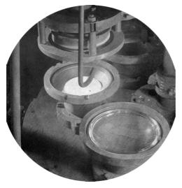
Above: The moulds in action, with a finished lens at the front. The pressed glass lenses bore no identification marks apart from the Lucas brand name.
